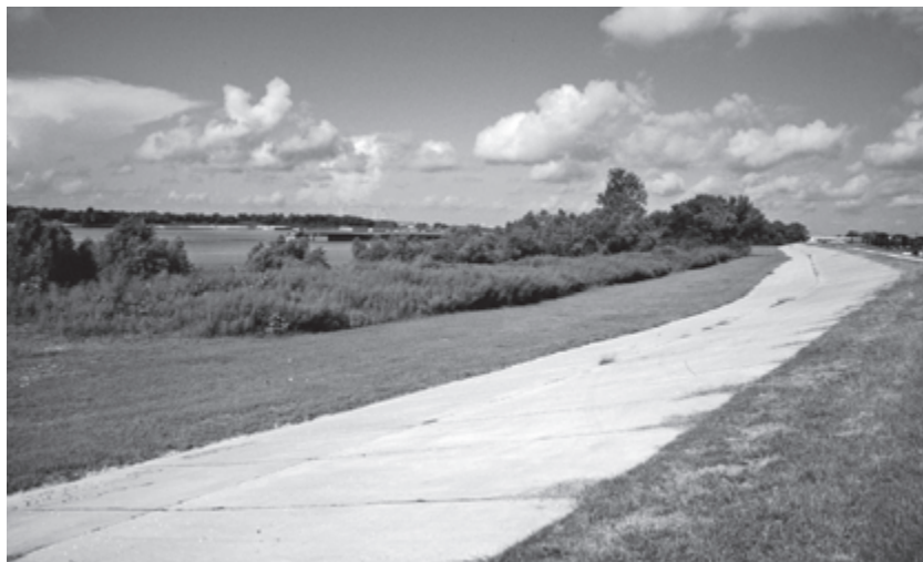
Fig. 3. A typical artificial levee along the Mississippi, with concrete erosion protection on the river face of the silt bank.
