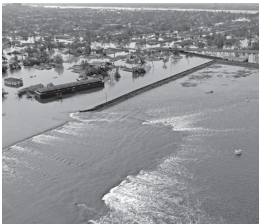
Fig. 9. Floodwater pouring through the broken levee beside the Industrial Canal. (Photo by FEMA)
