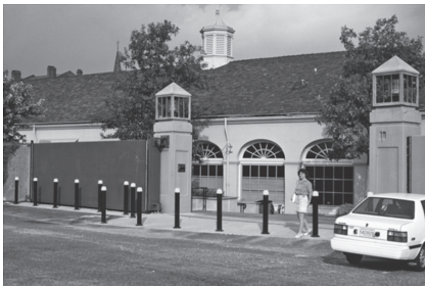
Fig. 4. Floodwall on top of the Mississippi levee in central New Orleans, with its gate open to allow access to a car park that is not used in flood times.
